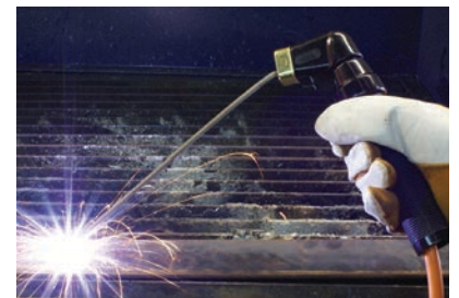
5) Strike the electrode against the work piece to create and arc and hold the electrode steady to maintain the arc
