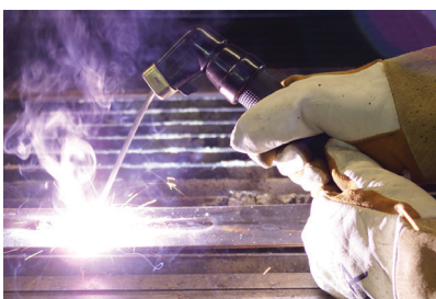
(6) Hold the electrode slightly above the work maintaining the arc while travelling at an even speed.
