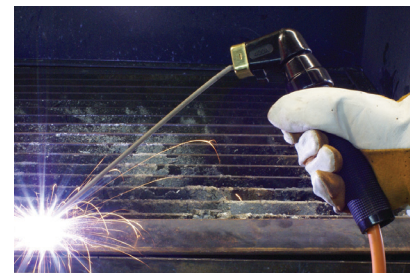
(5) Strike the electrode against the work piece to create and arc and hold the electrode steady to maintain the arc
